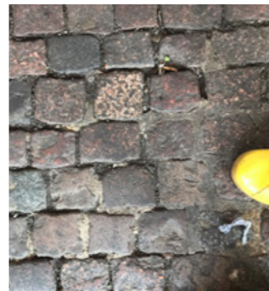
Staggered bond (square setts)
