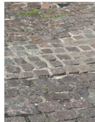
Stack bond (Square setts) limited use
