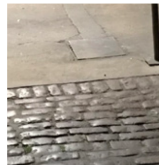
Rotated rectangular setts
