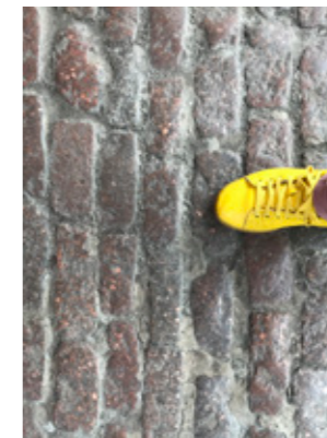
Staggered bond (rectangular setts)
