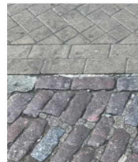
Rotated rectangular setts
