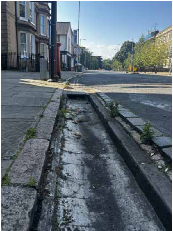
Hobson's conduit exposed runnel along Trumpington Street
