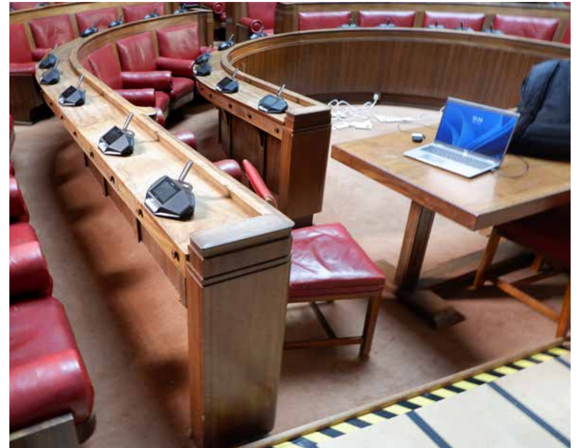
Council Chamber with exposed cabling and hazard tape evident. Floor level changes visible and restricted access into and around the fixed furniture arrangement.
