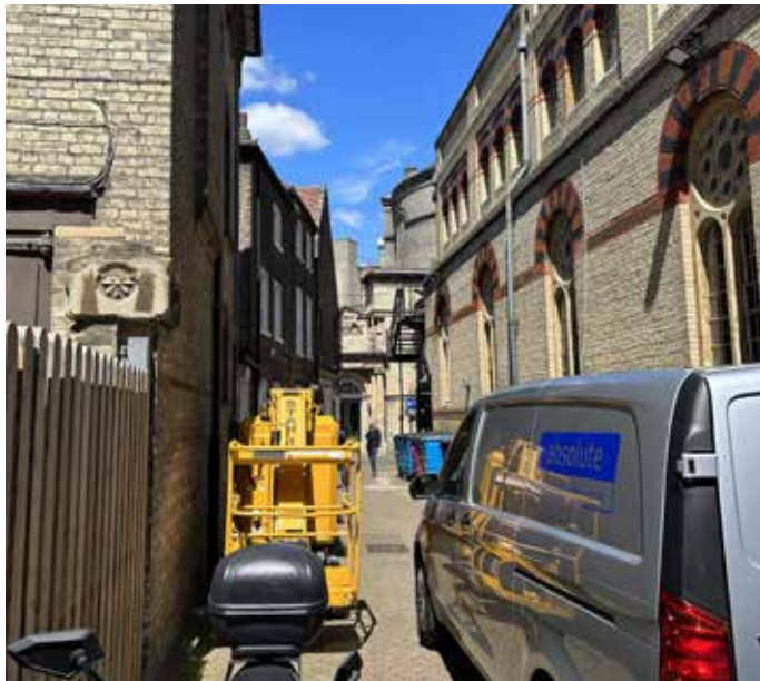
Equipment & Vehicle Congestion
