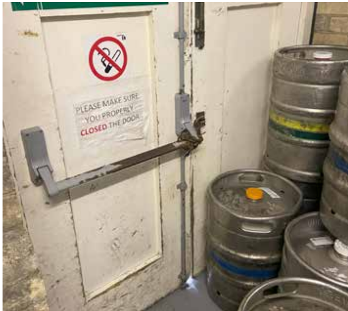
Lack of Storage
