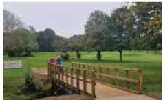
Bridge at key crossing
