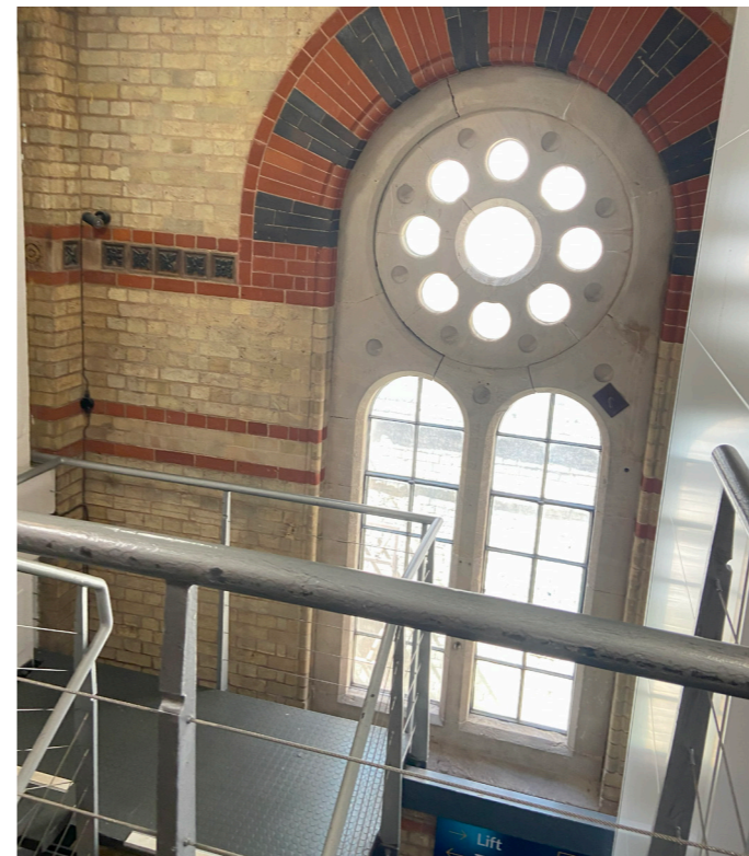
Mezzanine Level Stair
