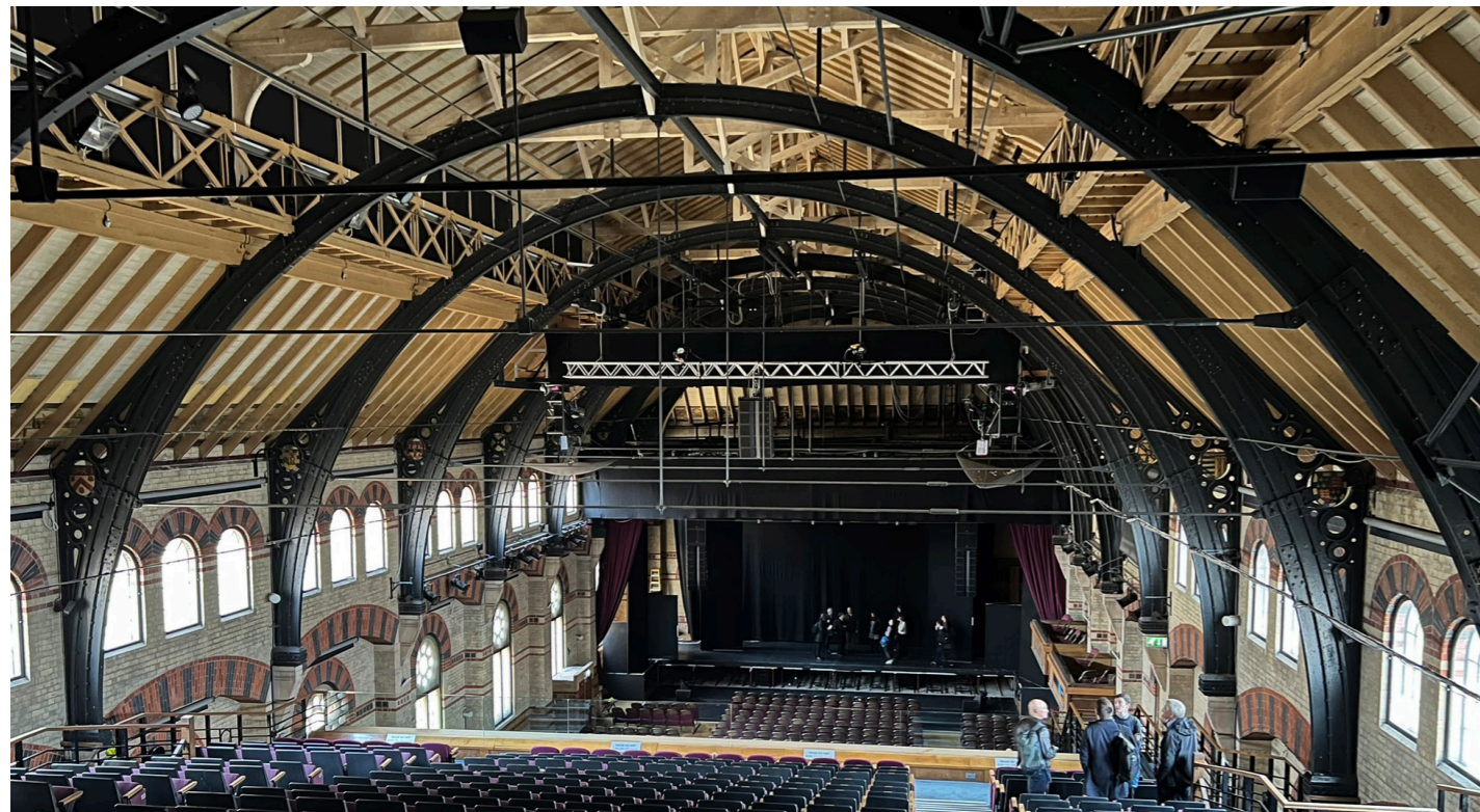
Top of raked seating view
