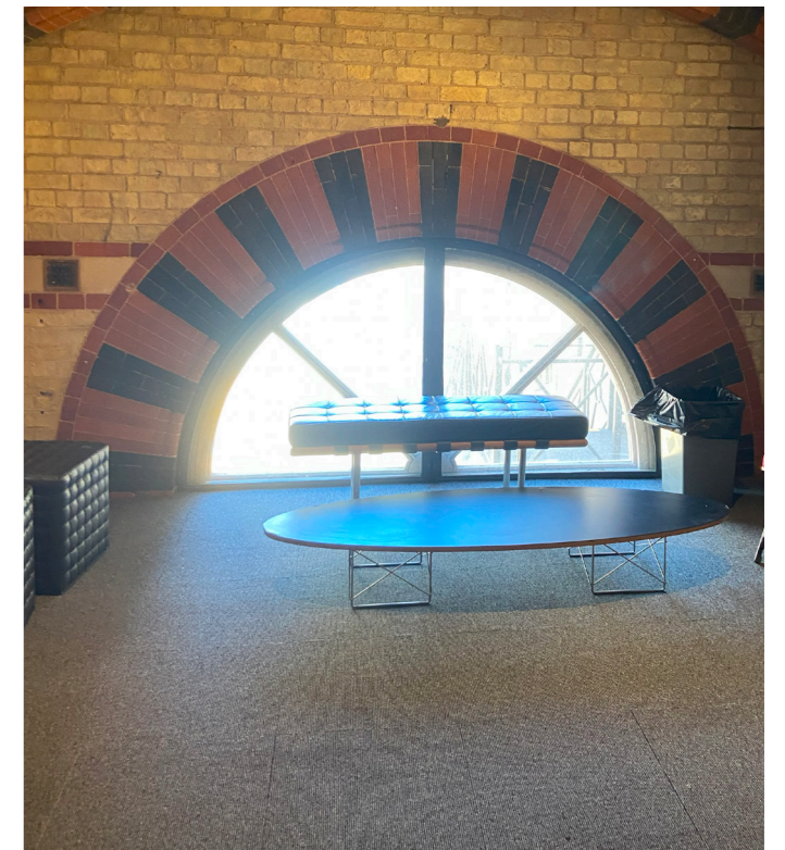
St. Johns Bar arched brickwork
