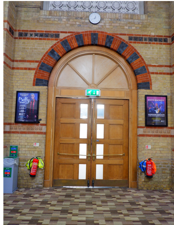
Front entrance double doors
