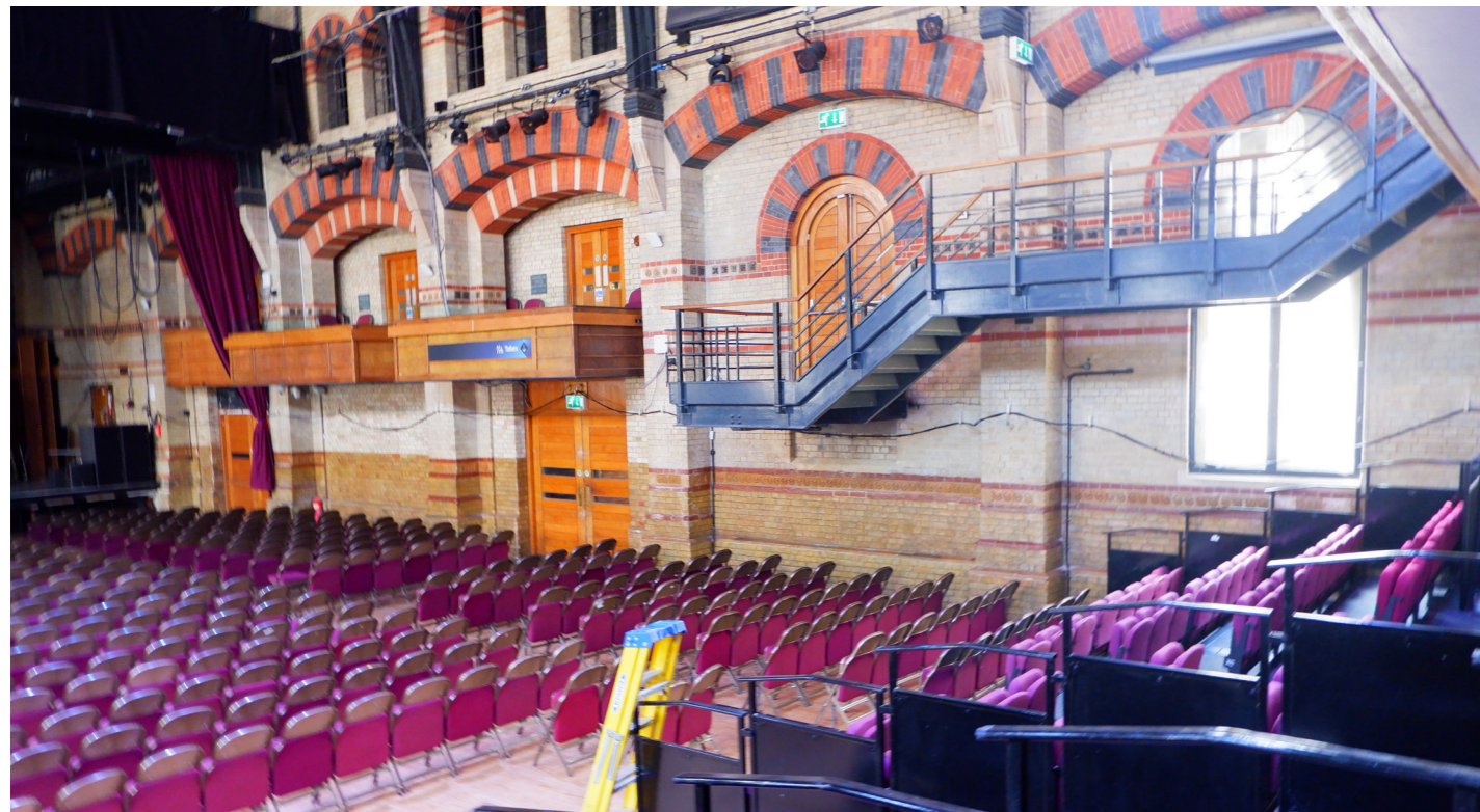
Fire escape stair from Auditorium
