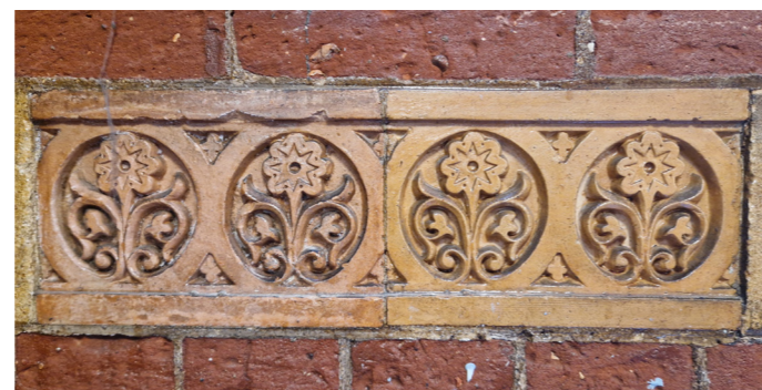
Decorative external tiling
