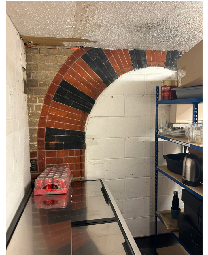
Blocked up arched brickwork
