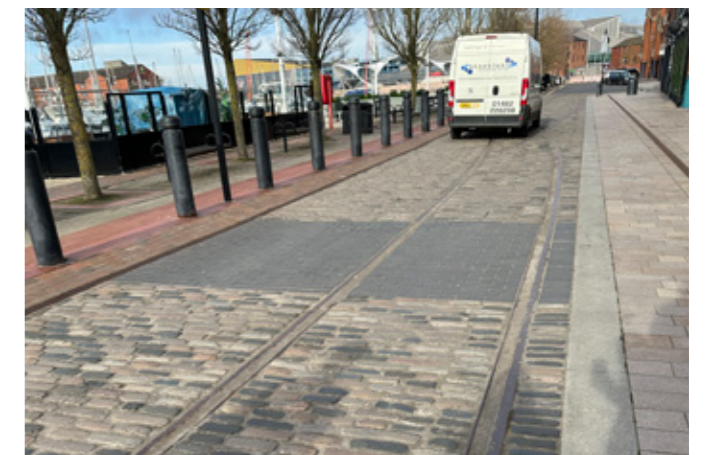
↑ Historic setts within a level, accessible surface
