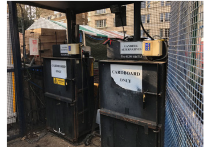
↑ Market Square: Cardboard waste compressor (understood to currently be out of action)
