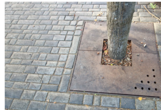
↑ Industrial style tree pits
