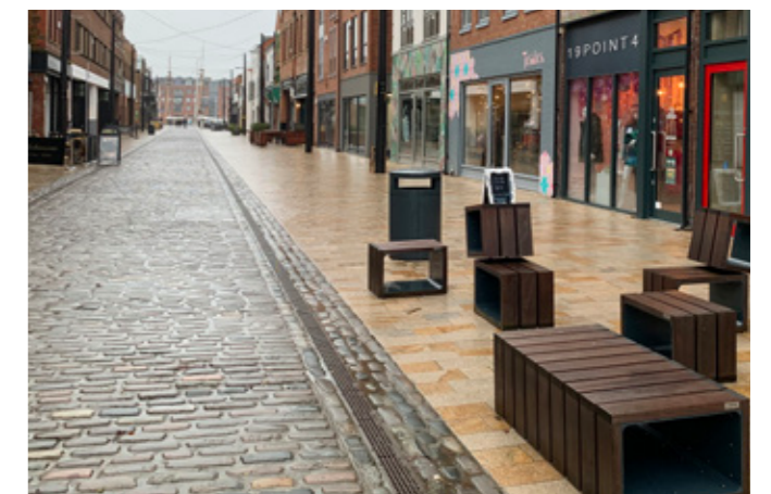
↑ The carriageway is clearly distinguished by materials
