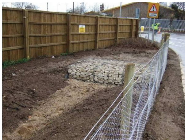
Gabion inlet shortly after construction (see diagram above)
