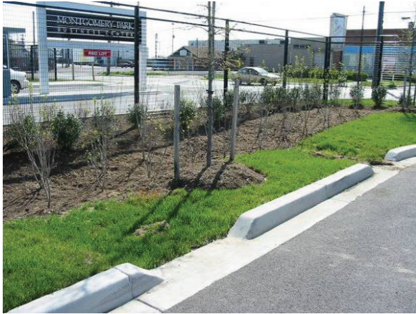
Dropped kerb inlet to rain garden
