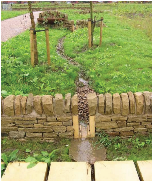
Swale detail where it passes through a wall in a park, Sheffield
