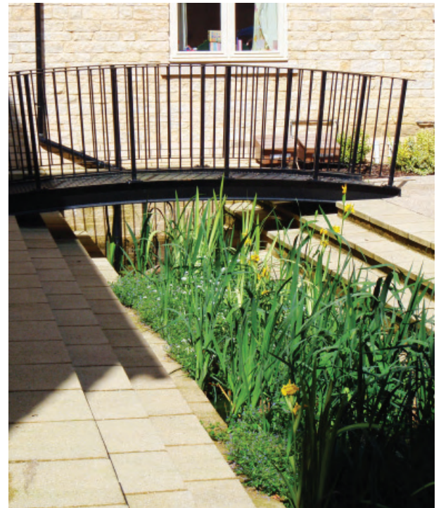
High quality SUDS for a high density development were achieved by early consideration in the design process – Stamford
