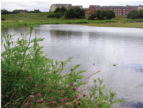
SUDS in Sheffield during the 2007 floods – there was no flooding from this system and it effectively managed runoff in rainfall that far exceeded the design storm, because it had a management train.
