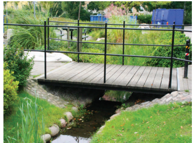
Low flow channel through public park in Malmö.
