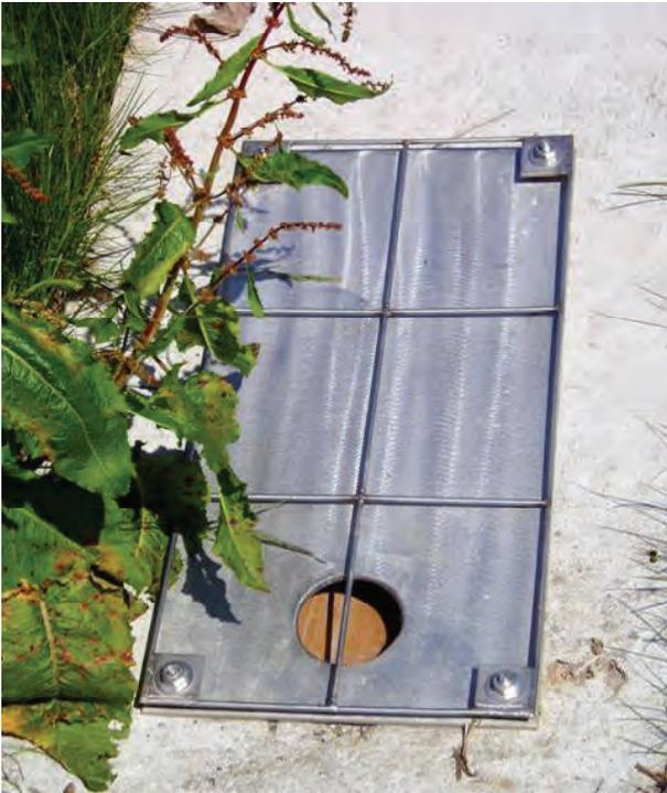
*Orifice control to a basin located on the surface so that it is easily accessible*
