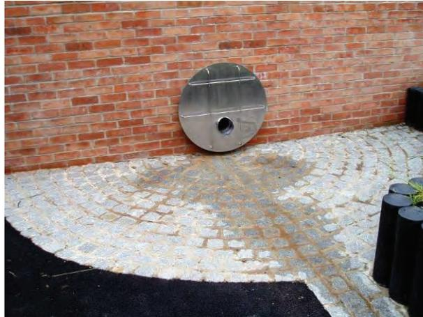
*Stainless steel outlet leading to a surface rill*
