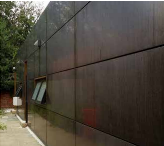
Concealed panel joints example
