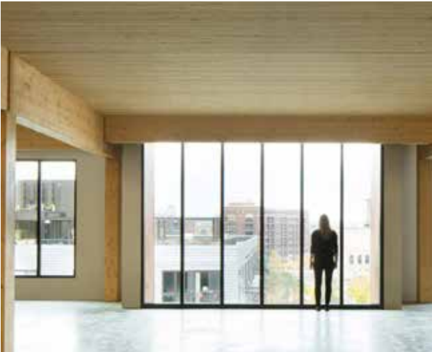
Exposed CLT soffit and Glulam column example
