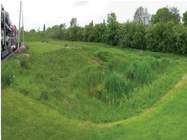
Retention basin with a wetland bottom, motorway service area, M42
