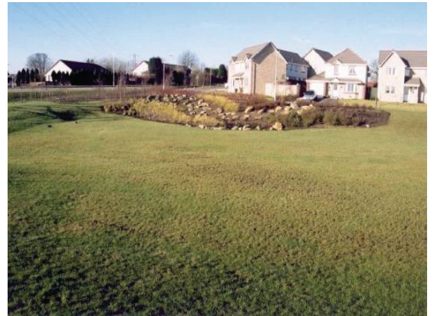
Shallow retention basin with easy access for maintenance, forming part of the public open space for the development
