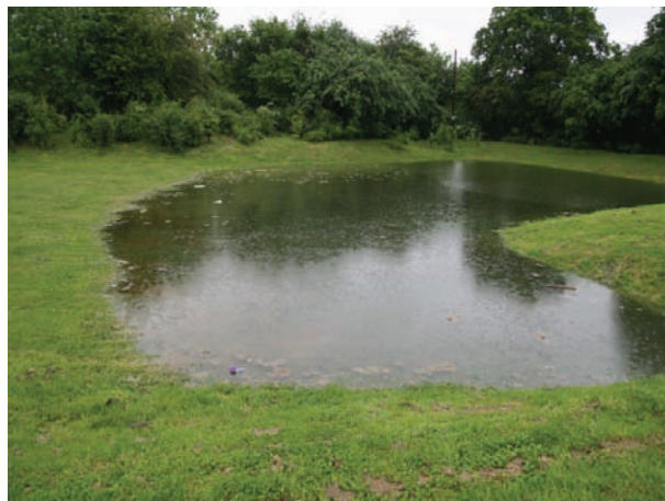
Infiltration basin during rainfall in a housing development. The basin is normally dry and contains water occasionally, Petersfield
