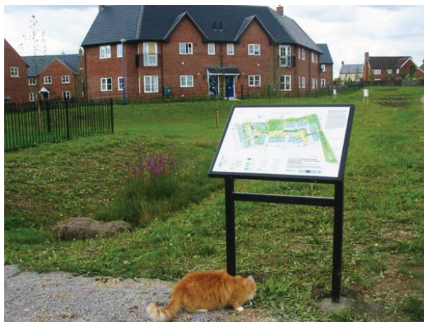
Basin in a housing development with an information board to explain its purpose to residents, Cambourne
