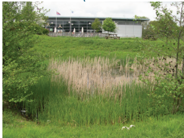
SUDS pond/wetland in a motorway service area showing different zones, Hopwood Service Area, M42
