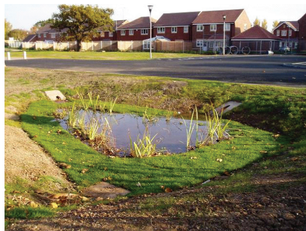
Turf used as erosion control in a pond, Worcestershire
