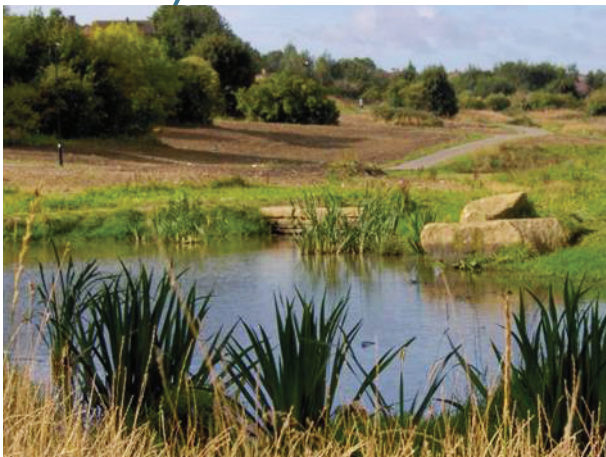
SUDS pond in a public park designed for biodiversity with shallow side slopes and safety bench, Sheffield
